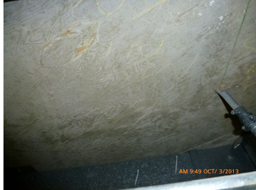
Reinforced Concrete Roof Deck
