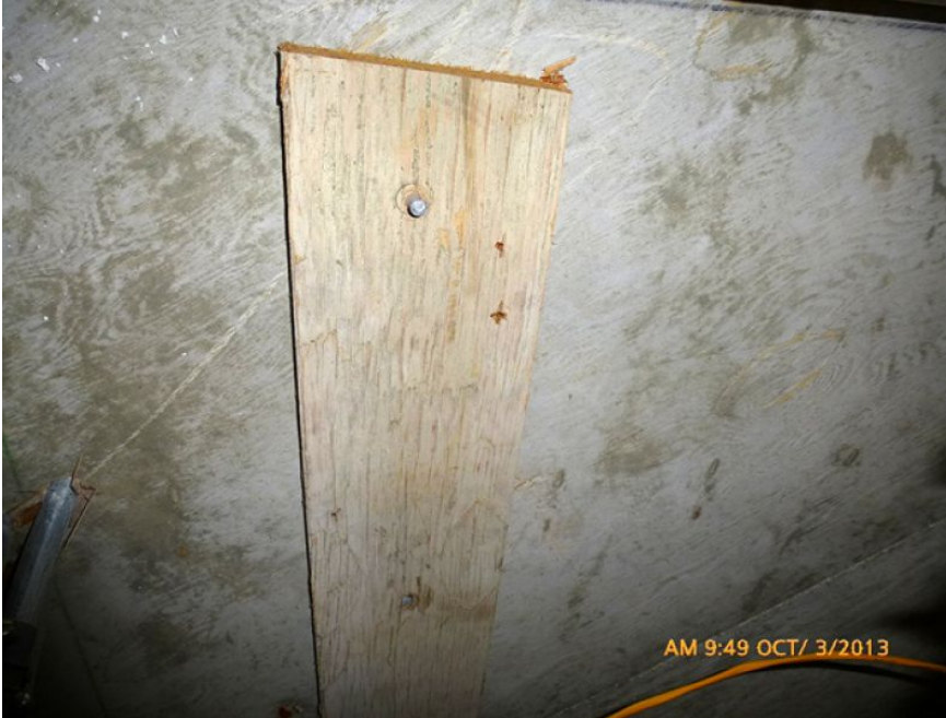
Reinforced Concrete Roof Deck
